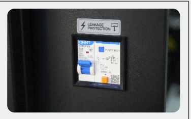
POWER LEAKAGE PROTECTION UNIT
